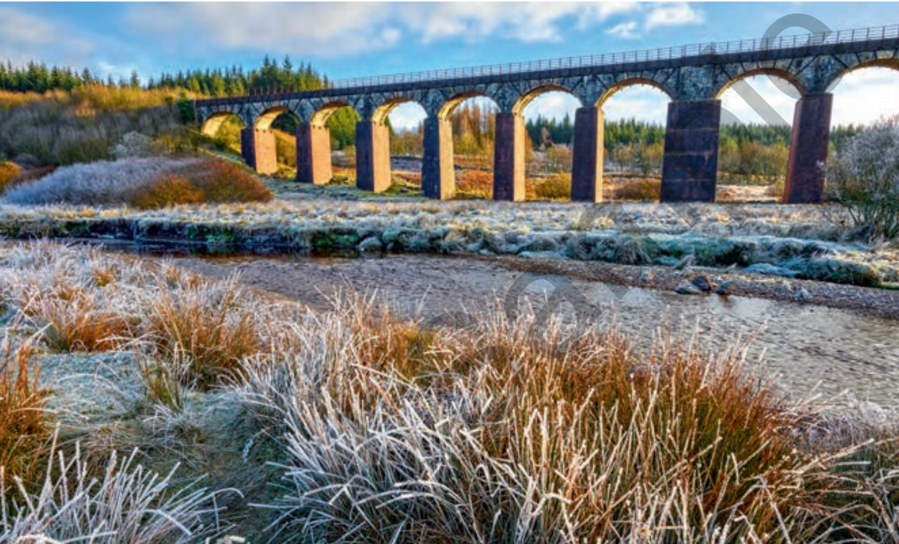
Big Water of Fleet Viaduct, Dumfries & Galloway
